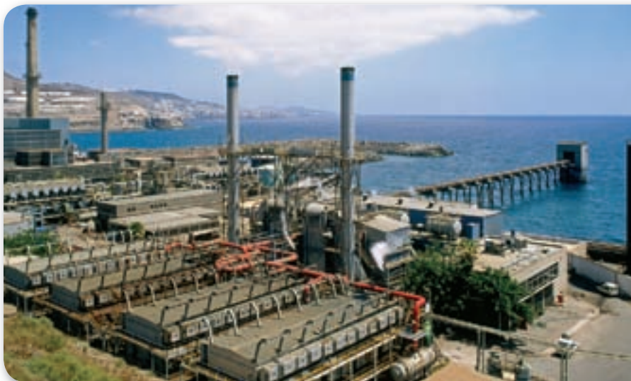
■ Figure 24.21 Desalination can be accomplished using several different methods. One method, called distillation, removes salt by boiling the water. Another process involves pumping the water through a filtration system to remove the salt. In some places water is desalinated in plants like this one.
