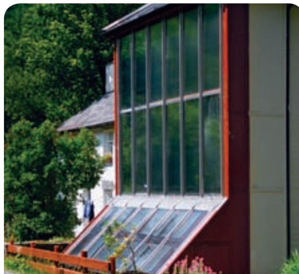
Passive solar heating
